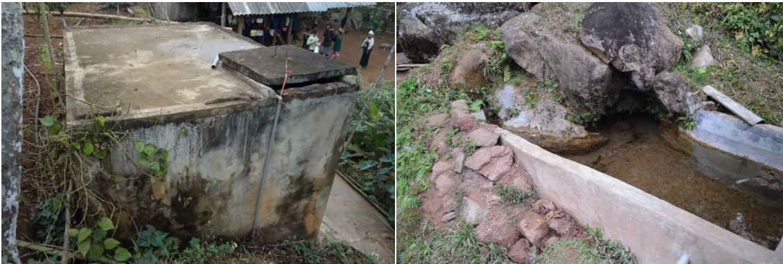
Figure 1. An example of a common water tank observed in many regions worldwide (a receiving water tank installed adjacent to a sugarcane farm ( Left ) and a rice field ( Right ) in Hòa-Binh Province, Vietnam) (Photo: Negishi).
