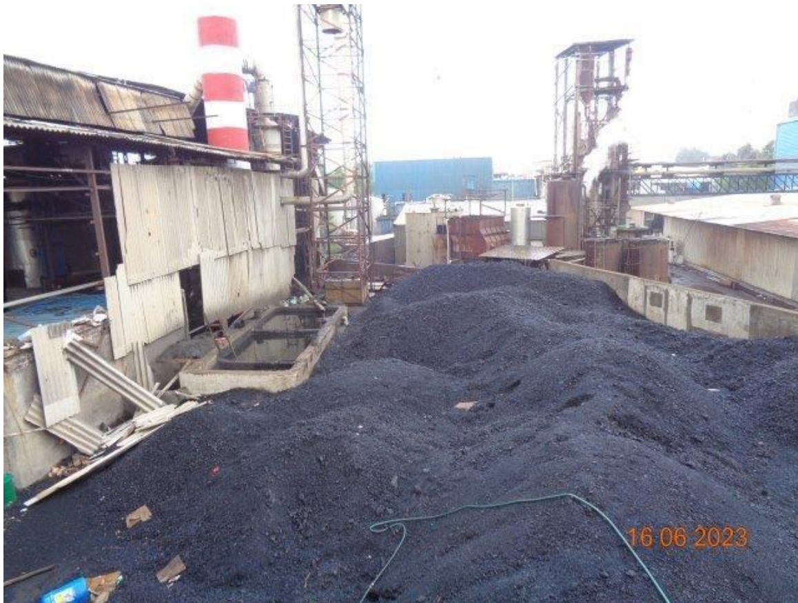
Figure 2. Coal combustion residues not disposed safely.
