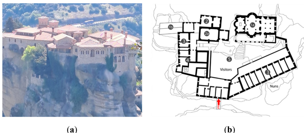
Figure 7. (a) Spaces built on top of rock cavities; (b) Spaces built on top of rock cavities plan (author archive and [5]).
