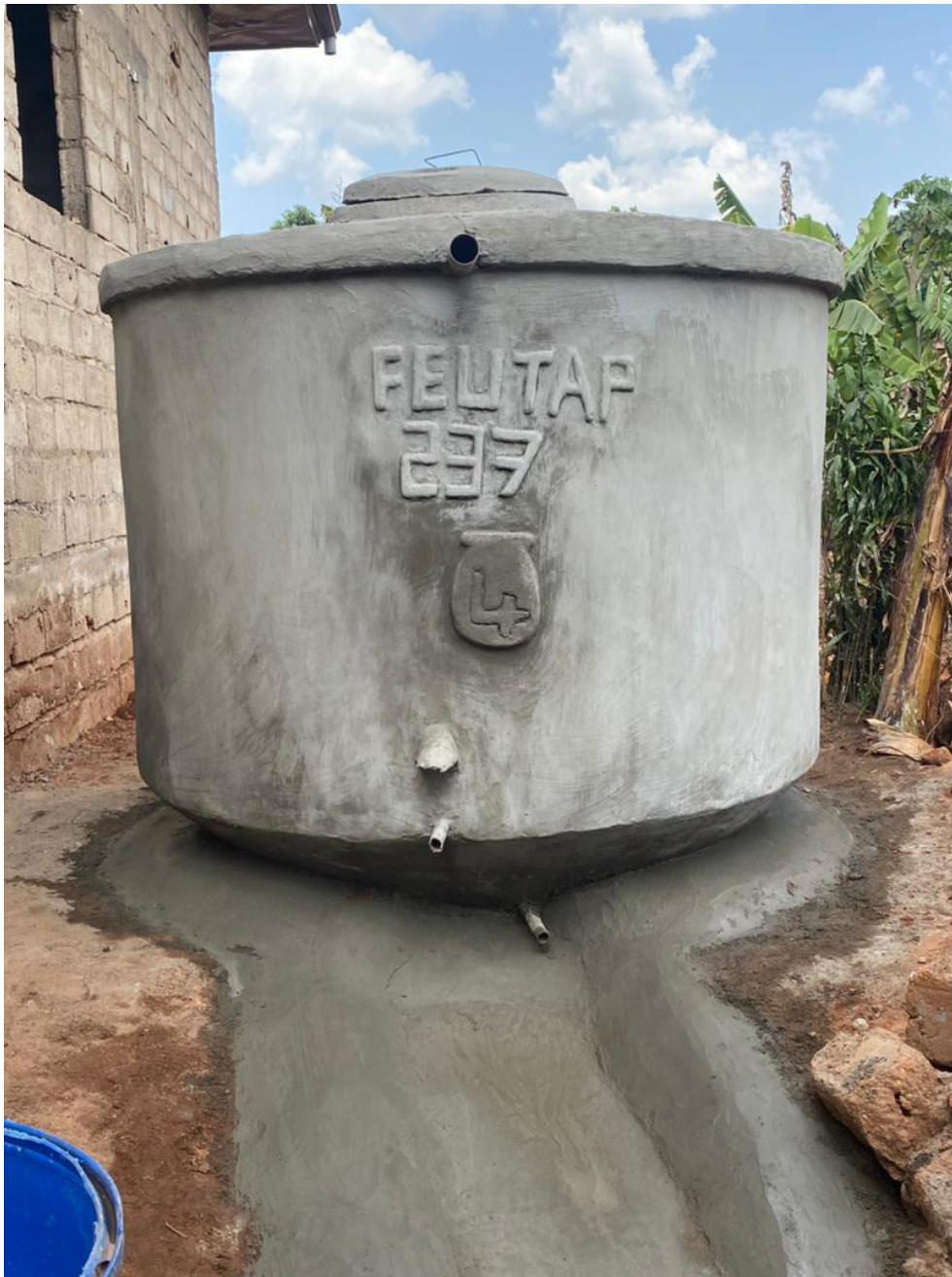
Figure 8. Photograph of an Akkerman Calabash recently constructed in Feutap (Bangangté, Cameroon). Photo taken by Vanick Fansou (January 2026).
