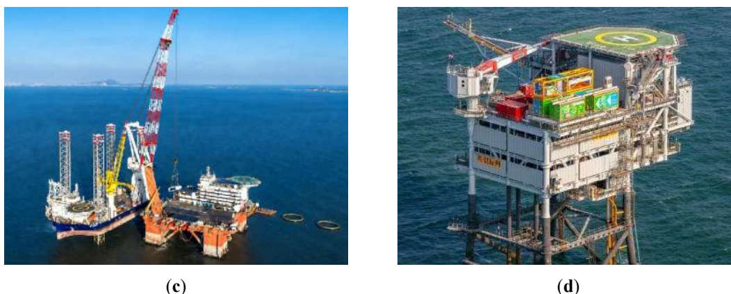
Figure 4. Engineering case: (a) Dongfu-1 platform; (b) Shenneng Hainan CZ2; (c) Offshore Hydrogen-Ammonia-Methanol Integrated Project in Yantai, Shandong. (d) Dutch PosHYdon demonstration project.
